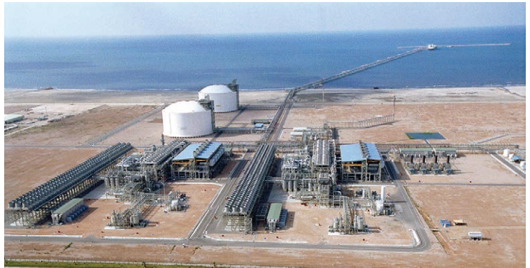
It is planned to export some gas from the proposed Leviathan field to BG Group's LNG plant at Idku, Egypt Source: BG Group
